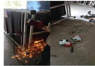
Gambar 22. Pergantian Roda Rack
