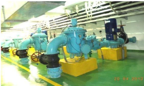
Gambar 7. *Cooling water pump (CWP)*
