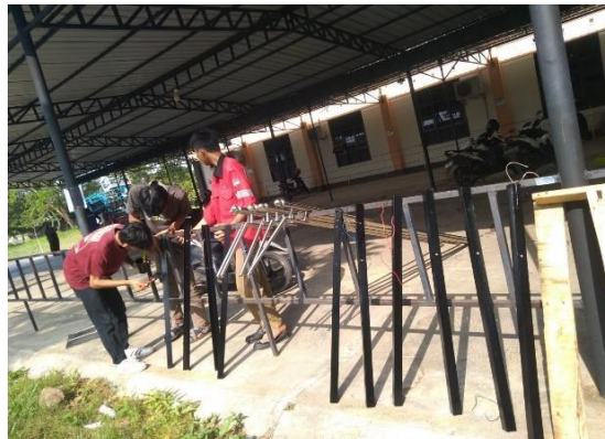
Gambar 8. Proses Pengecatan Besi Hollow
